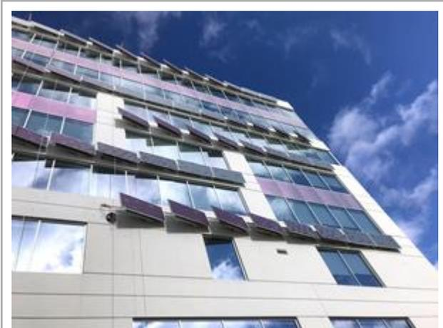
MoZaic East (by Ackerberg Group) is a building-integrated photovoltaic (BIPB) commercial solar project in Minneapolis, MN. Solar design and installation: All Energy Solar; inverter technology" Enphase Energy; solar module overlays: SolarSkin from Sistine Solar
