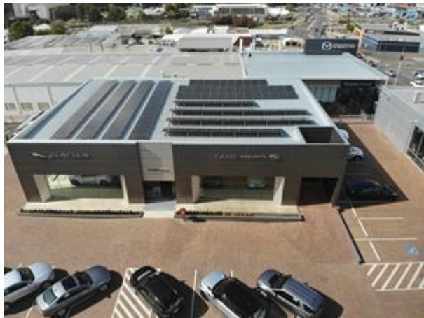
Excel Power deployed a 50 kW Enphase microinverter-based system for Wippells Autos, a Jaguar and Land Rover dealership in Toowoomba City, Queensland
