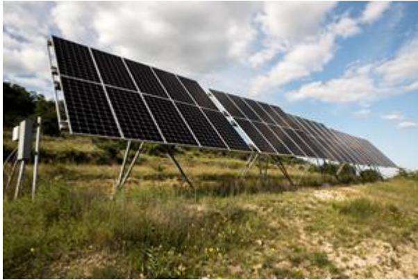
The solar system donated by Enphase, Mission Solar, and IES Texas solar was mounted on decommissioned satellite dish mounts.
